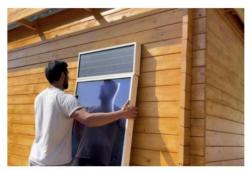
SunAéro can be installed vertically or horizontally on the exterior facade of a house facing the sun (ideally facing south, or south-east, south-west) via modular panels which are fixed to the partition by mechanical fixing with quick fasteners. With its "Plug & Play" system, installation is very simple: once you have chosen the room you want to heat, simply drill 4 holes on the outside of the front of the room to attach the panel.
